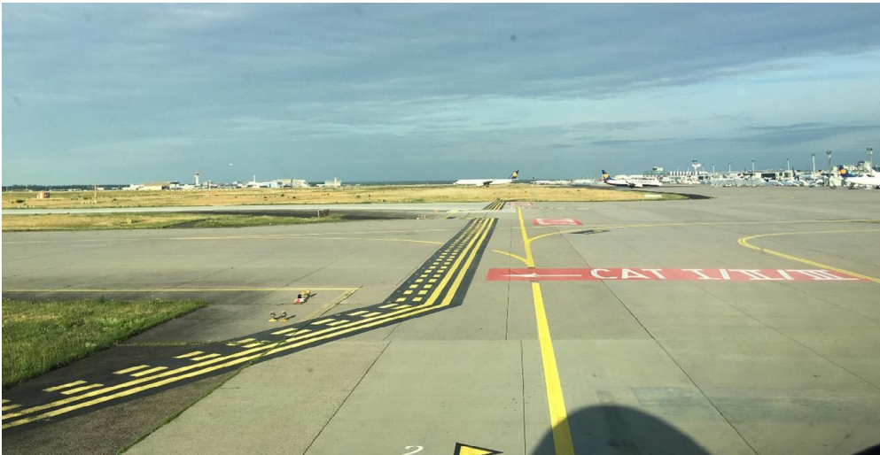
View from Twy L and the junction with Twy U (facing west).
